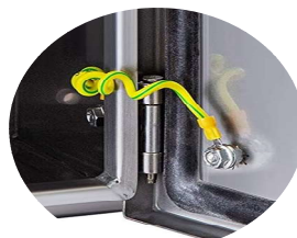
Door earthed to the enclosure
